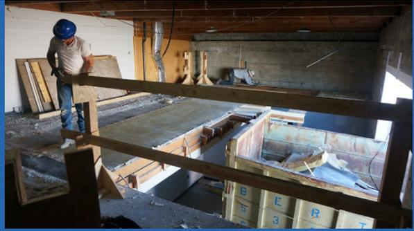
We're closer to completion on our new, extra large operations door. This will accommodate larger capacity cranes so we can move bigger motors into the building with ease. On the right, you can see demolition of the second story to accommodate the door.
