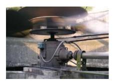
The most common solution for driving the fan in modern cooling towers utilizes an induction motor, driveshaft, disc couplings, guards and gearbox arrangements. Historically, this configuration resulted in high maintenance, vibration, noise levels and high energy consumption. For years, this has been the standard operating system for cooling towers...until now.
