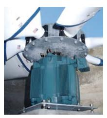
The Baldor • Reliance RPM AC Cooling Tower Direct Drive Motor mounts directly to the fan.
