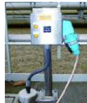
Decontactors simplify design, installation and maintenance of difficult to reach equipment such as submersible mixers or pumps.
